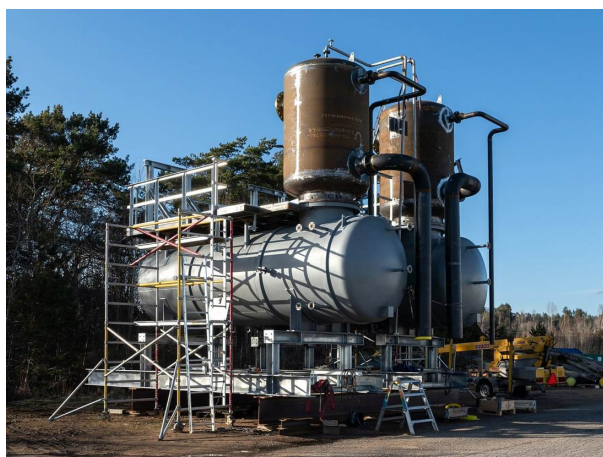
Photo: W.carter, Wikimedia Commons, CC0 – https://commons.wikimedia.org/wiki/File:Pressure_tanks_under_construction.jpg
