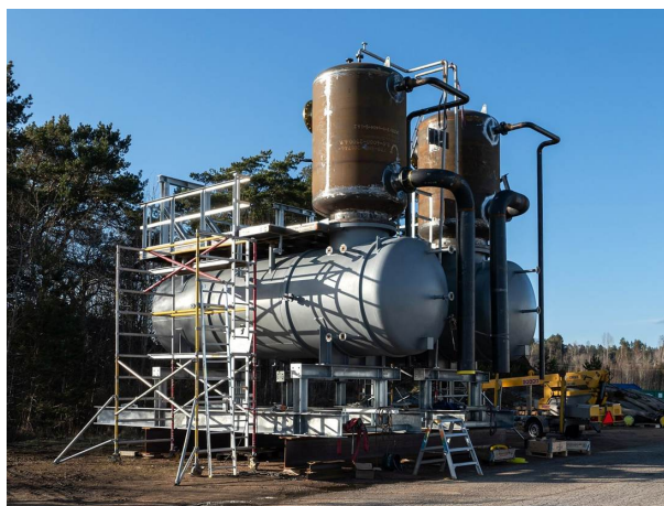
Photo: W.carter, Wikimedia Commons, CC0 – https://commons.wikimedia.org/wiki/File:Pressure_tanks_under_construction.jpg
